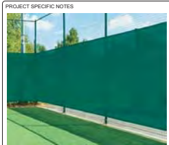
GREEN MESH PRIVACY SCREENING TO BE FIXED TO EXISTING POST & WIRE FENCING
