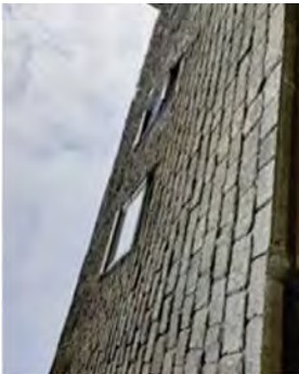
View on slate roof showing flush roof windows
