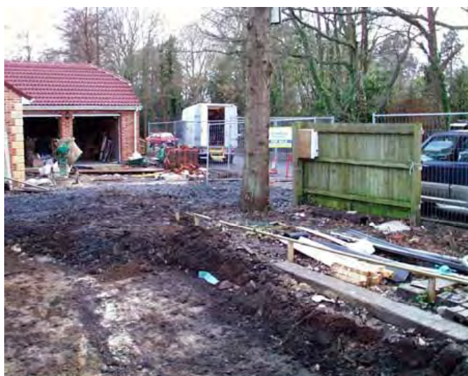
This tree has suffered both root damage and compaction damage due to vehicle movements and storage of materials. This tree is unlikely to survive.
