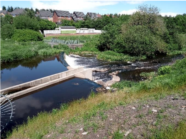
Plate A1.1 Kirkton Weir with in channel Larinier looking downstream
