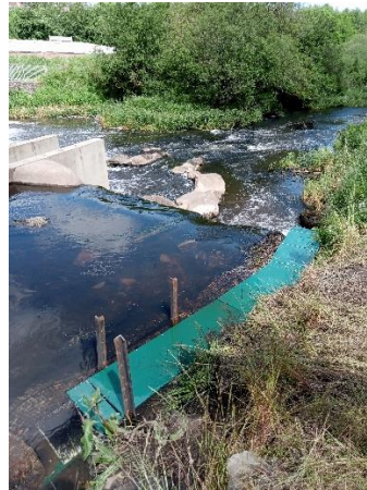
Plate A1.4 Eel pass at right-hand side of the channel (built in 2019)
