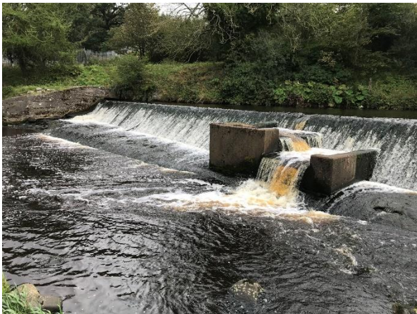
Plate B.1 Fish pass from island/ notch apparent
