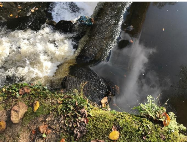
Plate A3.5 Notch in the weir at the top of the pass/ 29-10-19
