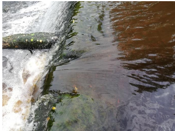
Plate B.2 Notch up close/ 2019 survey indicating it as measuring 0.6m wide and 0.13m deep
