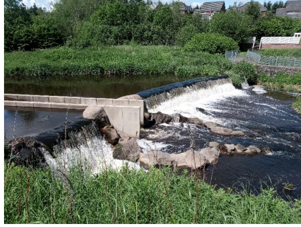
Plate A1.2 Kirkton Weir with in channel Larinier looking across the channel/ weir
