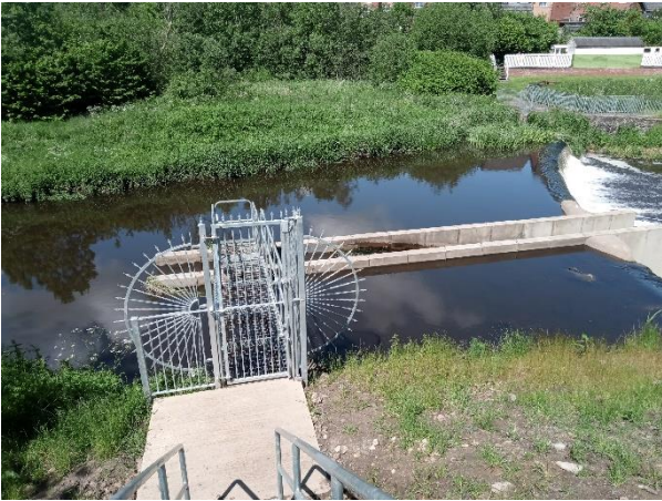
Plate A1.3 Access walkway and platform (added in 2018 after Larinier had been built)
