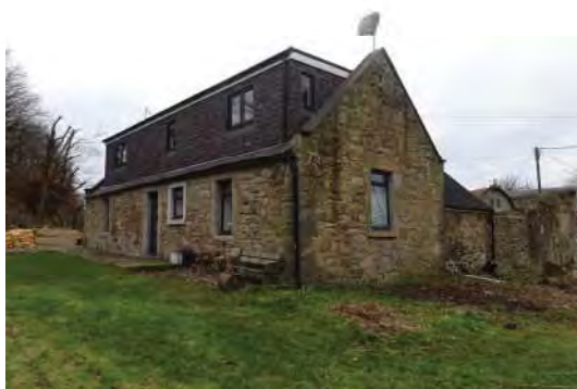
EXISTING VIEW OF REAR OF PROPERTY WHERE PROPOSED EXTENSION IS LOCATED
