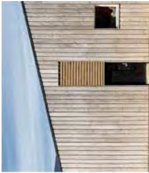
Natural timber cladding
