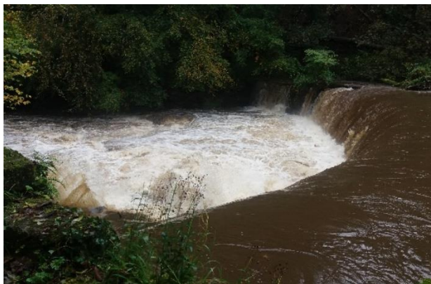
Plate A3.1 Hoghton Bottoms weir at time of high flow (fish pass to left submerged)/ 11-10-19
