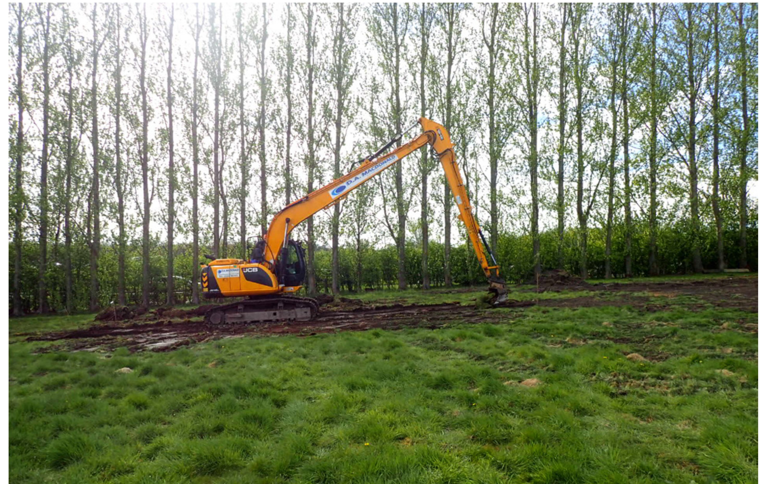
Ground investigation being carried out in a field to the north of Sheriffhall Roundabout
