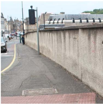
Poor quality blank rendered wall detracts from appearance of High Port and the arrival into the town from the south
