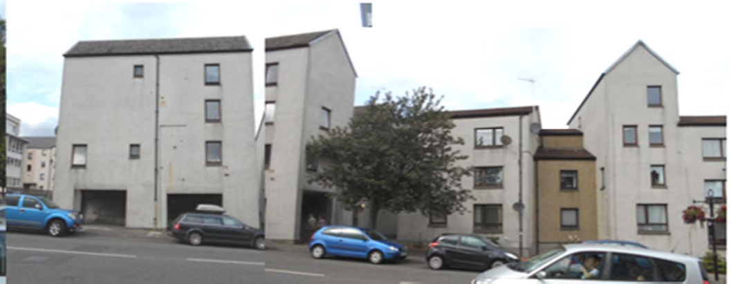
318-348 High Street: Flatted development circa 1975. Harled walls under a mix of slate and tiled roofs. Design includes colonnaded walkway over the pavement, historically a common feature of Linlithgow High Street largely lost by 1900.
