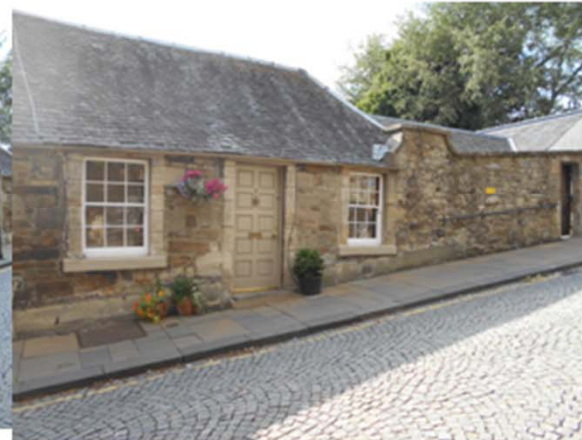
3 Kirkgate: Listed Grade B. Near symmetrical cottage. Circa 1700. Cream sandstone, slate roof. 12-pane sash and case windows. Good use of heritage colours.
